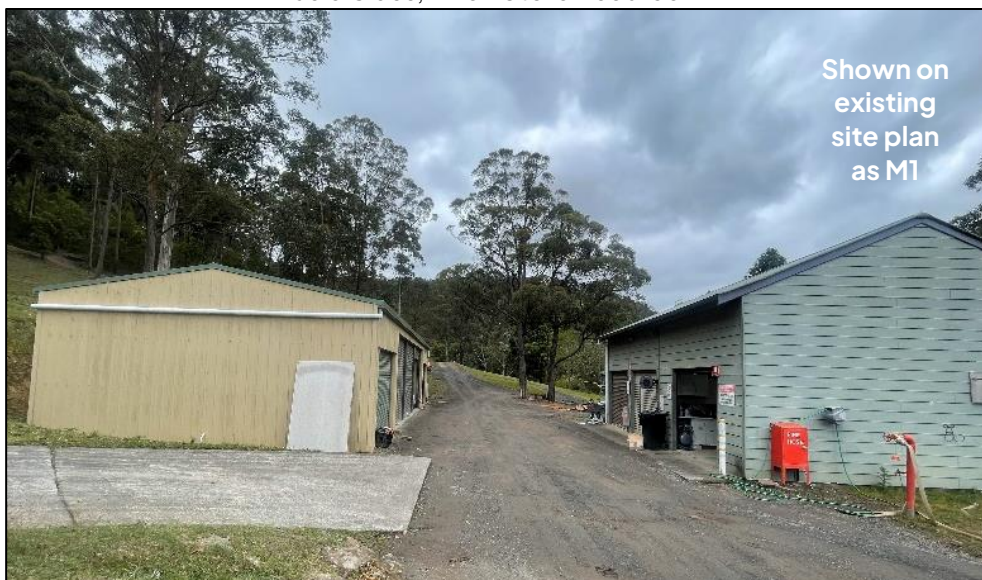
Figure 4 – Buildings on site to be demolished in Stage 1 – M1 Maintenance Facilities / Storage – source: AP
