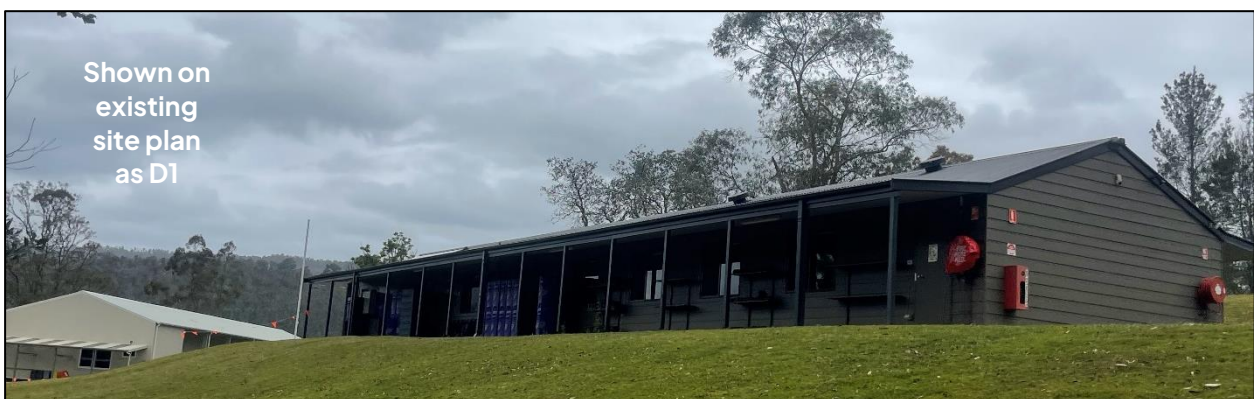
Figure 5 – Buildings on site to be demolished in Stage 1 – D2 Dormitory – source: AP
